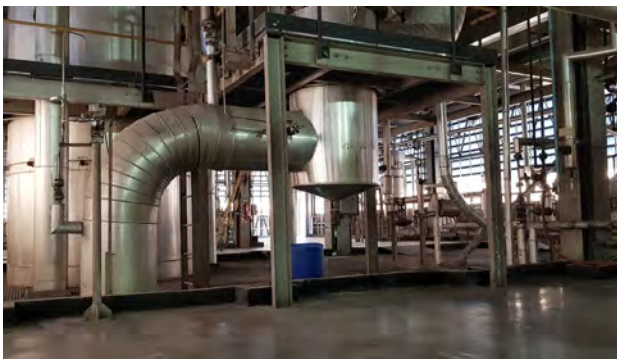
Steel structure assembly
